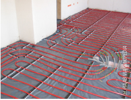
Raidant Hydronic System
