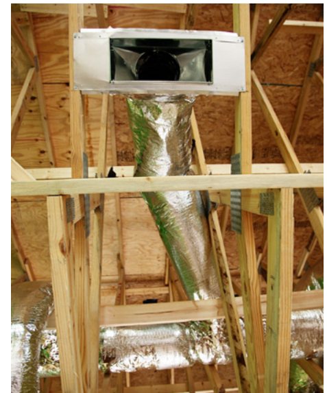
Ductwork in Attic
